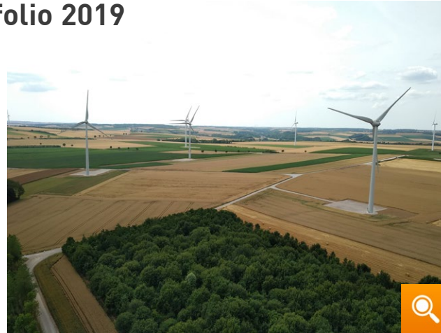
Audincthun wind farm commissioned in summer 2019 6 Enercon E-92/2.35 MW turbines – installed capacity 14.1 MW
