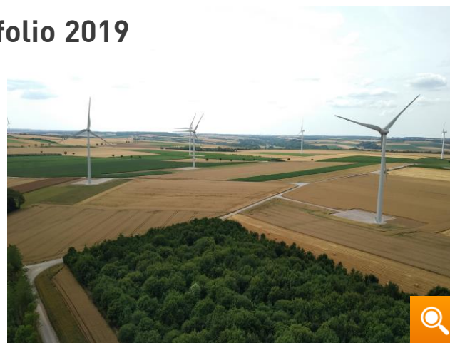
Audincthun wind farm commissioned in summer 2019 6 Enercon E-92/2.35 MW turbines – installed capacity 14.1 MW
