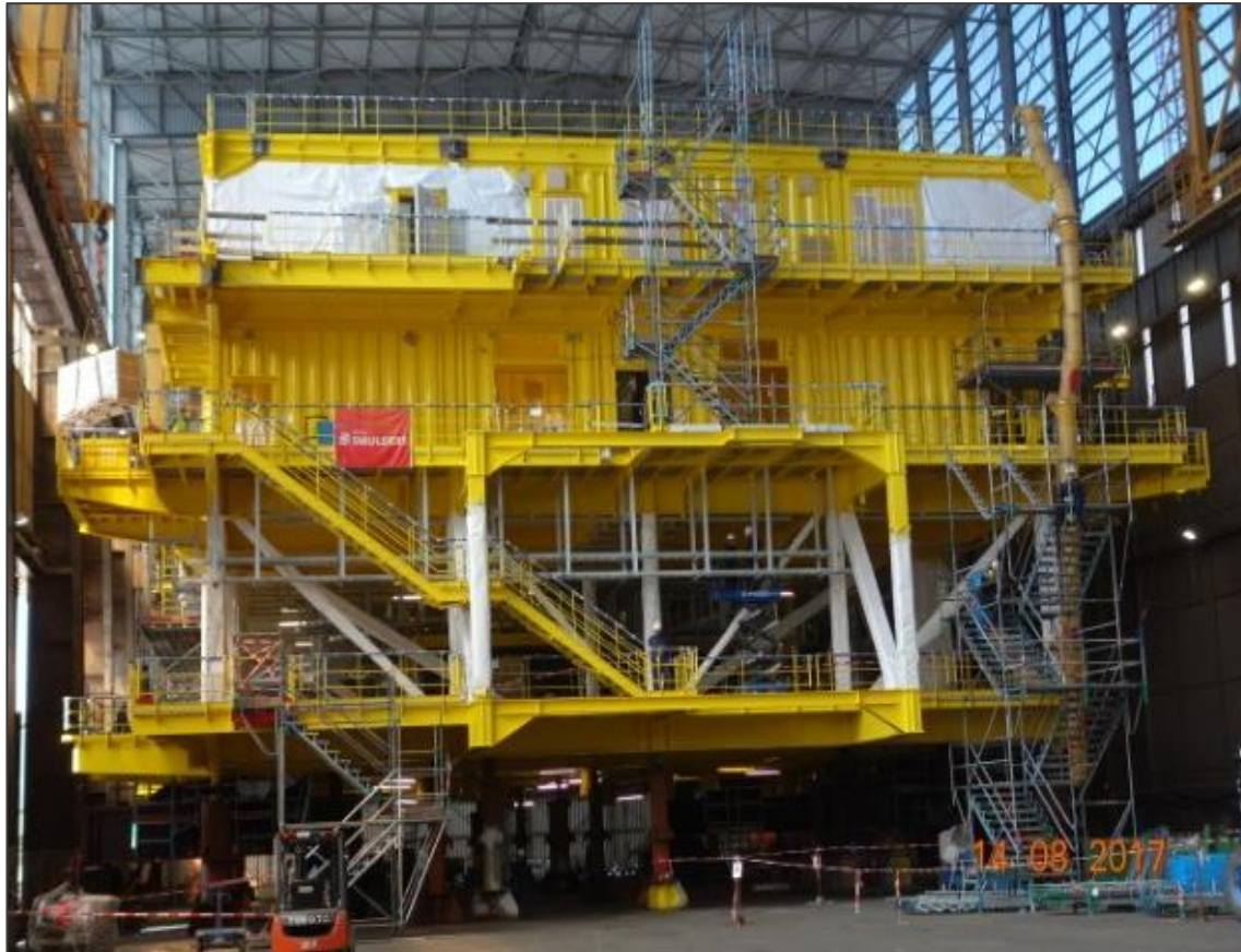
Offshore Substation (Hoboken, Belgium)
